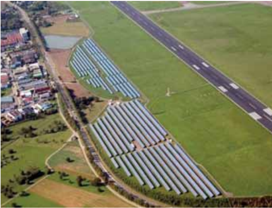
Saarbruecken Airport – Germany: PVPP over airport buffer zone
