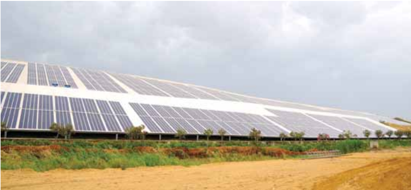
Solar Integrated T2 SolarRoof Membrane on a re-naturing landfill in Malagrotta, Italy
