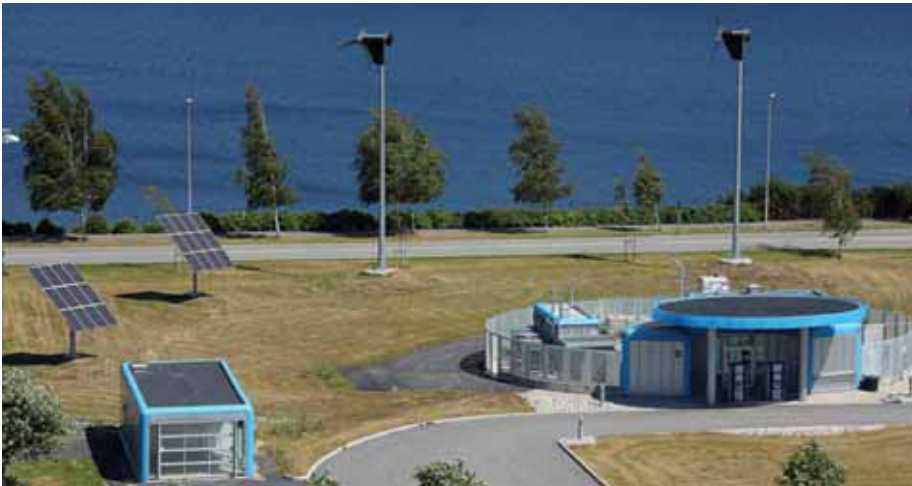
Statoil energy park, Porsgrunn, Norway. The demonstration site for the NEXPEL PEM-electrolyser.
