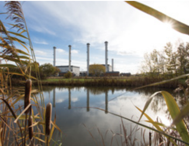
The natural gas storage at Rehden in Northern Germany is one of the largest natural gas storage facilities in Europe.
